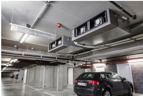
Heat exchanger installed in the garage, saving space
