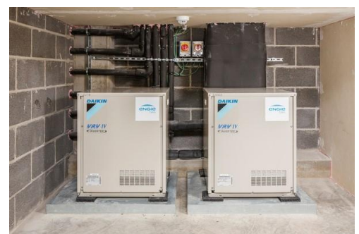
The compressor modules are highly compact and provide low-noise operation
