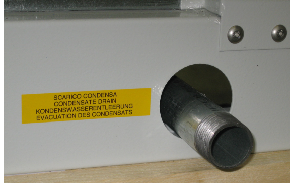
Fig. 9 Connection to the condensate collection tray
